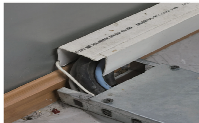
Fig.1 Power cables and signal cables installed in the same non-metal cable slot non-metal cable trays
